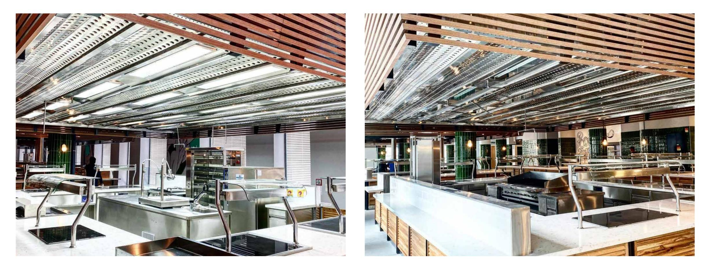
Project: "MAX" Head Quarter Front kitchen. Product: Ventilated Ceiling "ECONOVENT" series. Ventilated ceiling Area 152 m<sup>2</sup> [1636 ft<sup>2</sup>]. Project delivery year: 2020 Catering and high capacity kitchens 13
