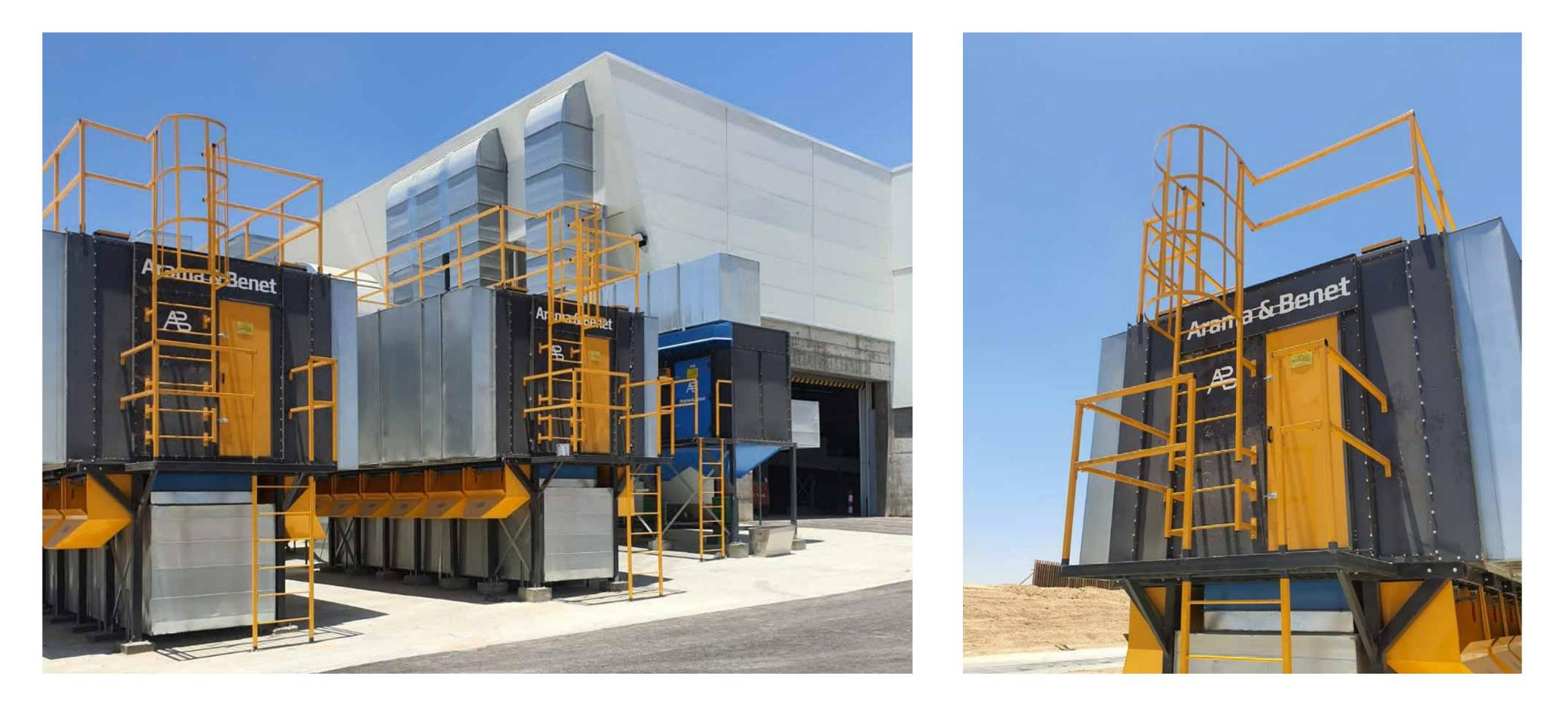
Project: "DUDAIM" Solid Waste Recycling Plant. Product: "Two stage Air Filtration System" Air Volume: 210.000 m<sup>3</sup>\h [123.500 CFM] Project delivery year: 2021 Industrial Air Filtration 82
