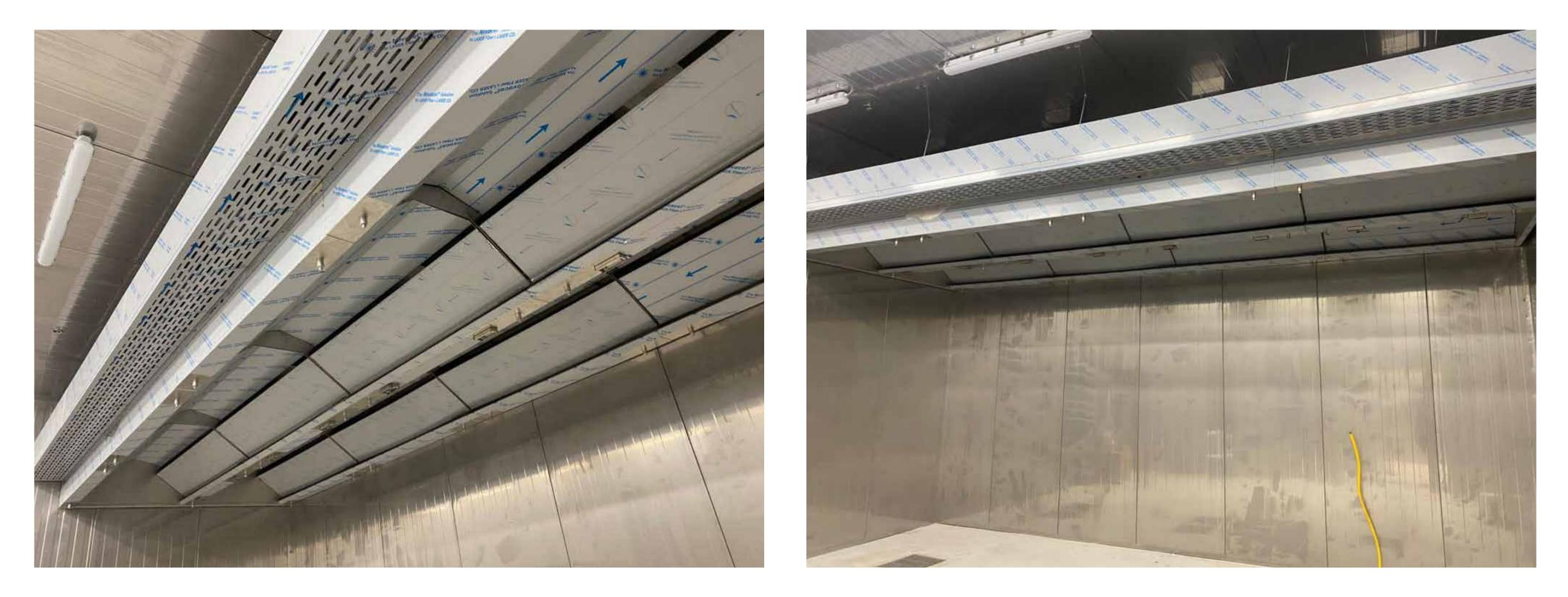
Project: Food Production Plant. Product: "CONDENSATION HOOD" with Water Condensate Anti-Drop construction. Project delivery year: 2021
